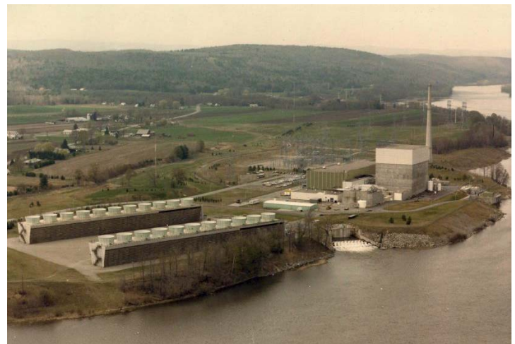
Vermont Yankee. The cylindrical structures in the foreground are the cooling towers, the boxy structure in the middle is the reactor building.
